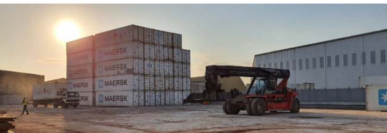
Grindrod's new intermodal facility in Durban
