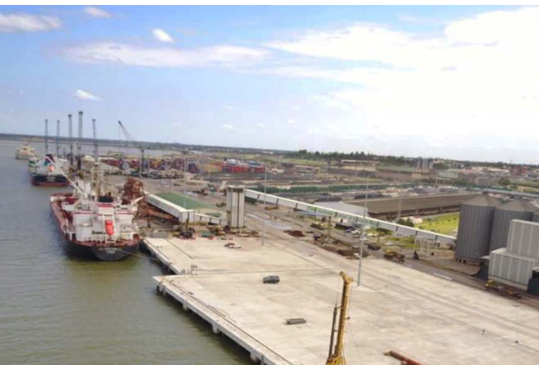
Upgrade of Berth 6, 7 and 8 port of Maputo
